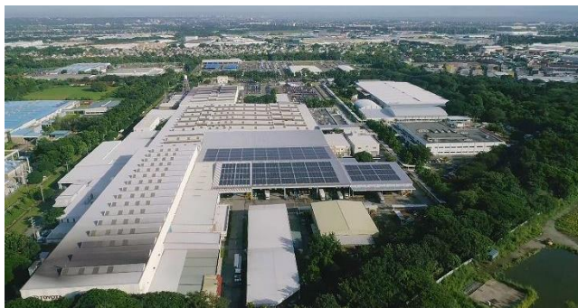
The 1-MW (Phase 1) of TMP Solar Array at its manufacturing plant in Santa Rosa City, Laguna was inaugurated in 2018
