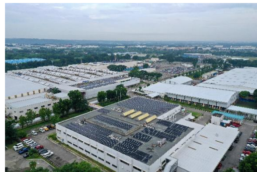
The 0.46-MW (Phase 2) expansion as seen on roofs of TMP's main building and administrative services center
